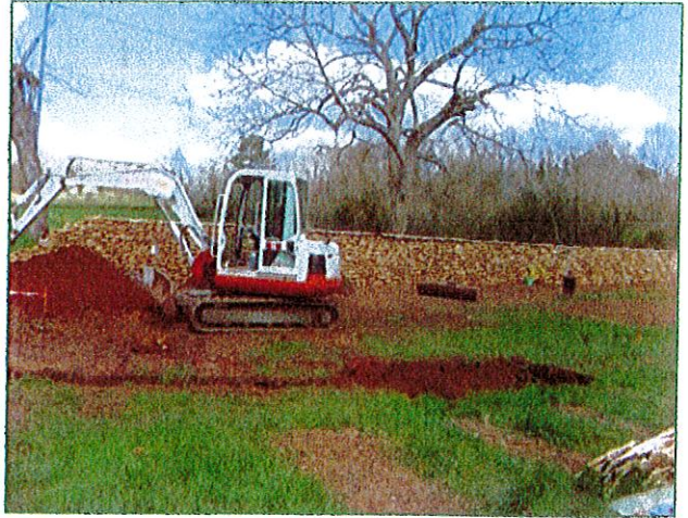
excavation of the septic tank
