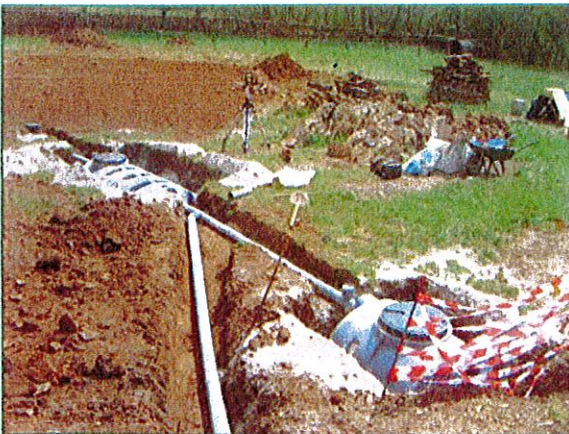
Connecting the septic tank
