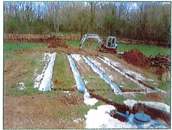
fitting the geotextile
