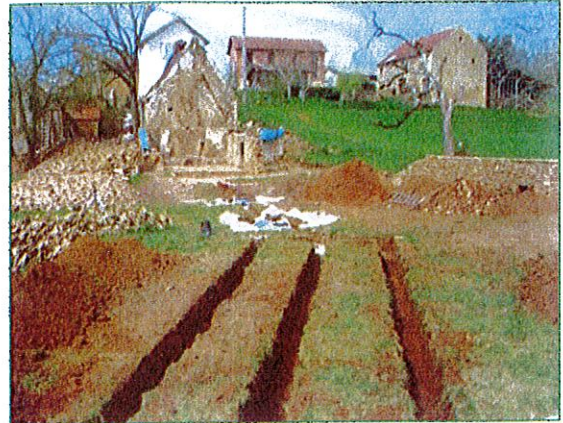
Excavation of the trenches of infiltration
