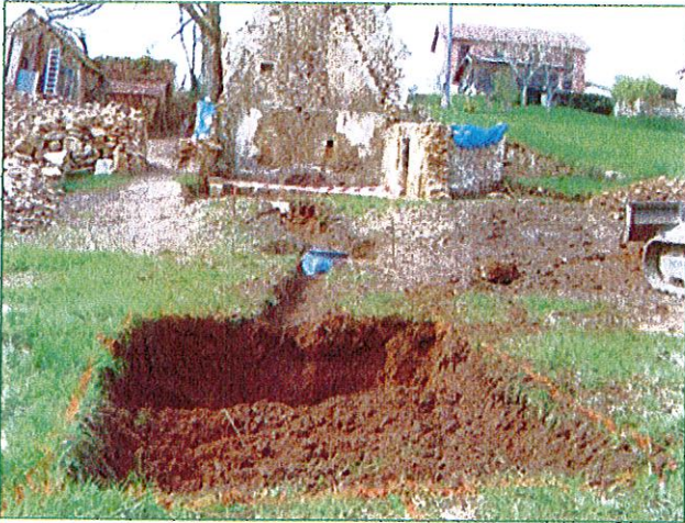
Excavation of the septic tank
