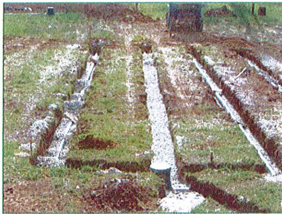
Filling up the trenches with gravel
