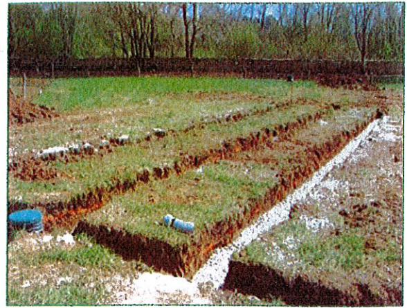
Filling up the trenches with gravel
