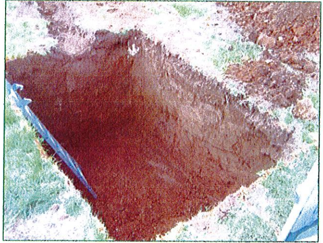
Excavation of the septic tank
