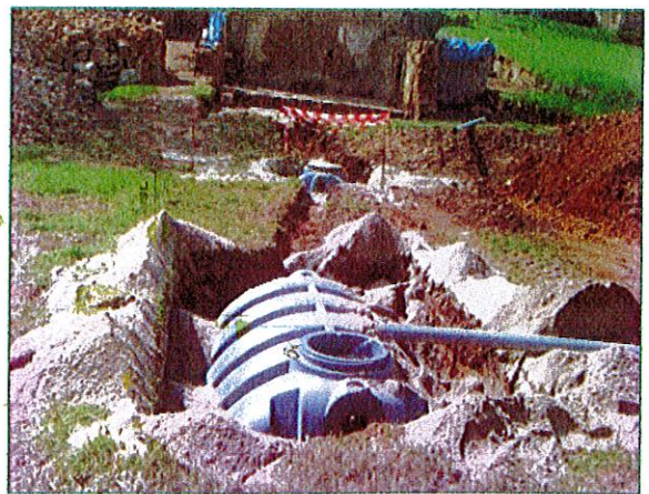
Filling up the septic tank with water
