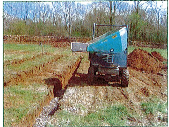
Filling up the trenches with gravel
