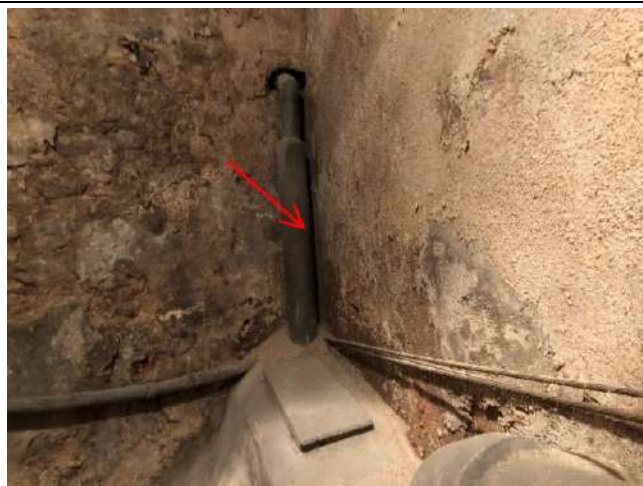
001 : fibre ciment Parties communes/Cave - garage
