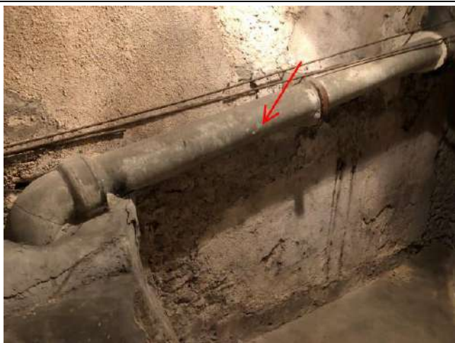
001 : fibre ciment Parties communes/Cave - garage
