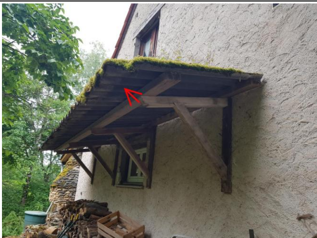
001 : fibre ciment Facade Sud
