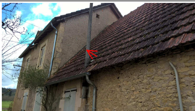
001 : amiante ciment Facade
